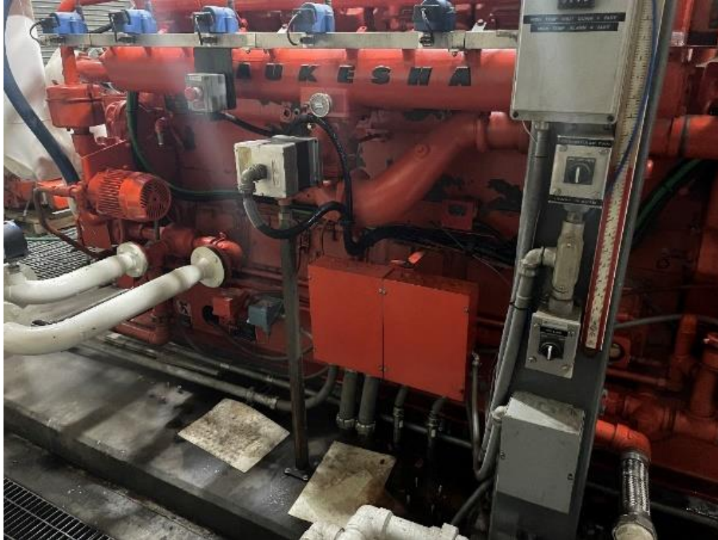
Old throttle body with a shaft through the block to sync the throttles
