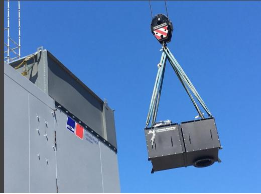
A Diesel Particulate Filter, or DPF for short, is a special filter on the exhaust system of a diesel standby generator. This filter removes particulates from the exhaust of a diesel engine and entraps them so that they do not pollute the air. This pollution control device is a critical component in your emergency backup generator and it is mandated, permitted, and controlled by the local AQMD in California.
