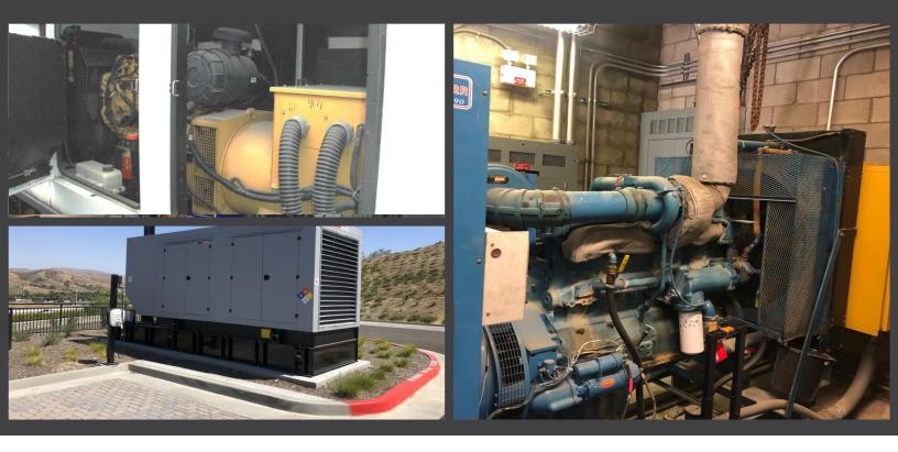
**4. FLUIDS** Contaminants - Among other contaminants, diesel tanks can become fouled by water or become corrupted by algae (which feeds off the diesel fuel). These fuel contaminants will cause the generator to fail to start because of substandard fuel or clogged fuel filters.
